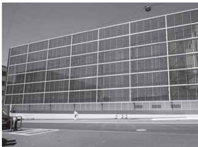
© CSEM: The bi-facial heterojunction facades in front of the CSEM clean rooms
