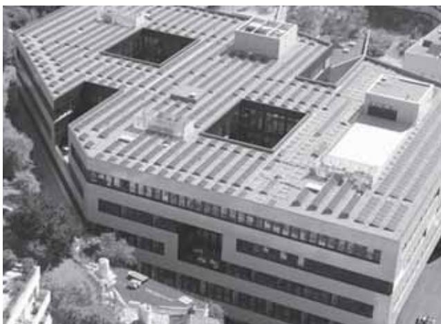
© EPFL: The EPFL Microcity building in Neuchâtel with its test PV power plants, next door to CSEM
